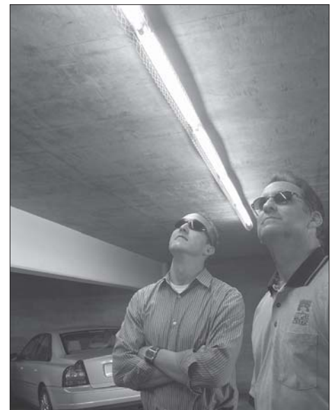
Public Services analyst Matt Huffaker, left, and Building Maintenance Supervisor Steve Schmidt inspect the new, energy-efficient lighting in the North Locust Street parking structure.
